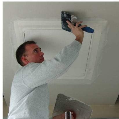
3. Smooth drywall tape and compound with a taping knife.
