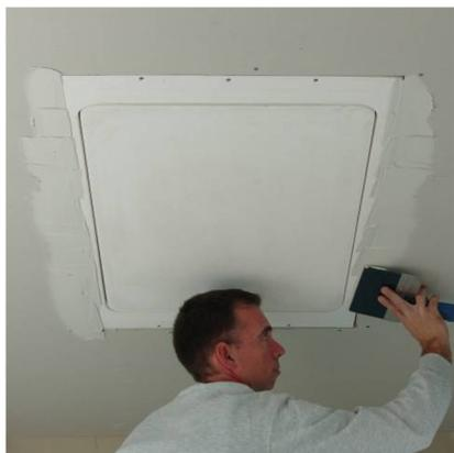
1. Apply drywall mud base, covering seams and screws.
